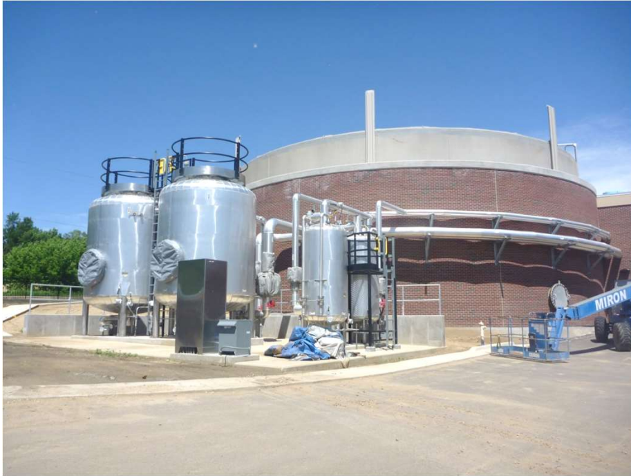
Media Based H 2 S and Siloxane Removal
