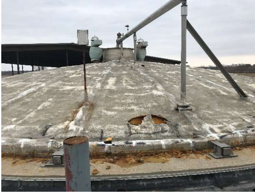
Rehabilitate and reinsulate newer stainless-steel covers
