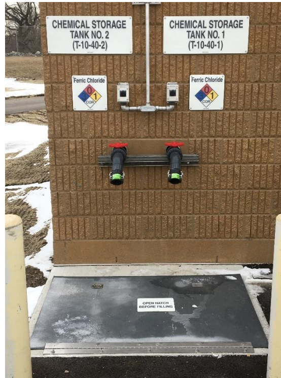
Tank fill with spill containment
