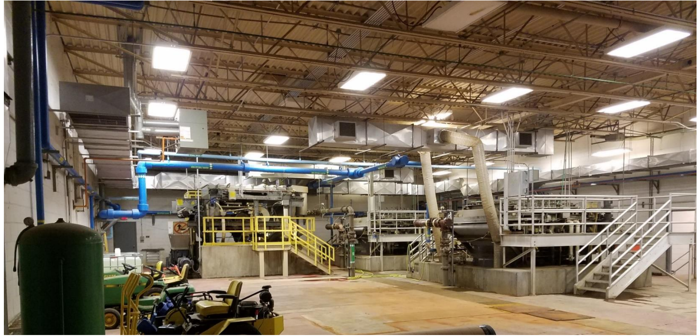
Existing dewatering equipment includes two belt filter presses installed in 1990 and one belt filter press installed in 2015
