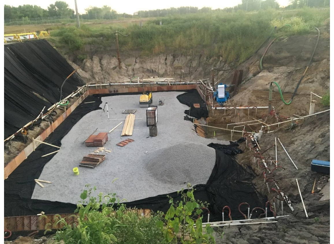
Progress photo – centrate tank excavation
