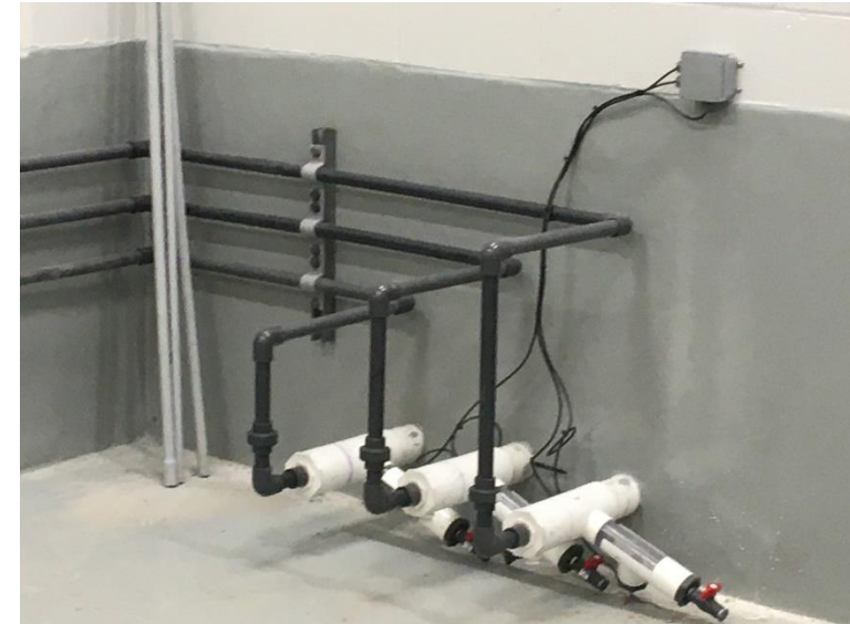
Containment and leak detection system
