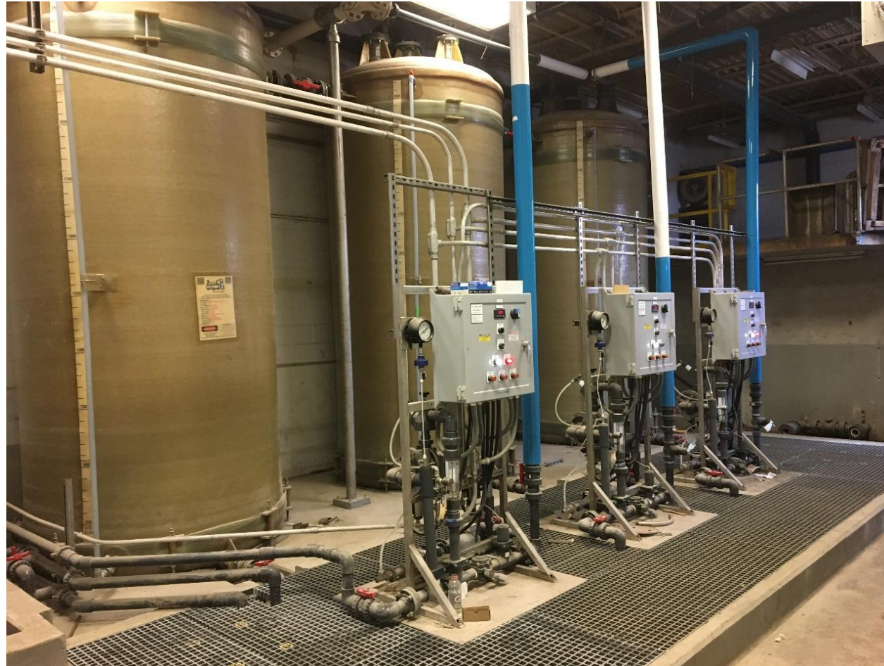
New polymer feed equipment and bulk storage tanks
