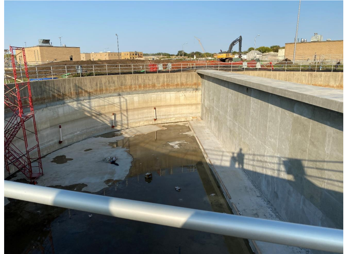
Progress photo – old equipment removed and divider wall installed
