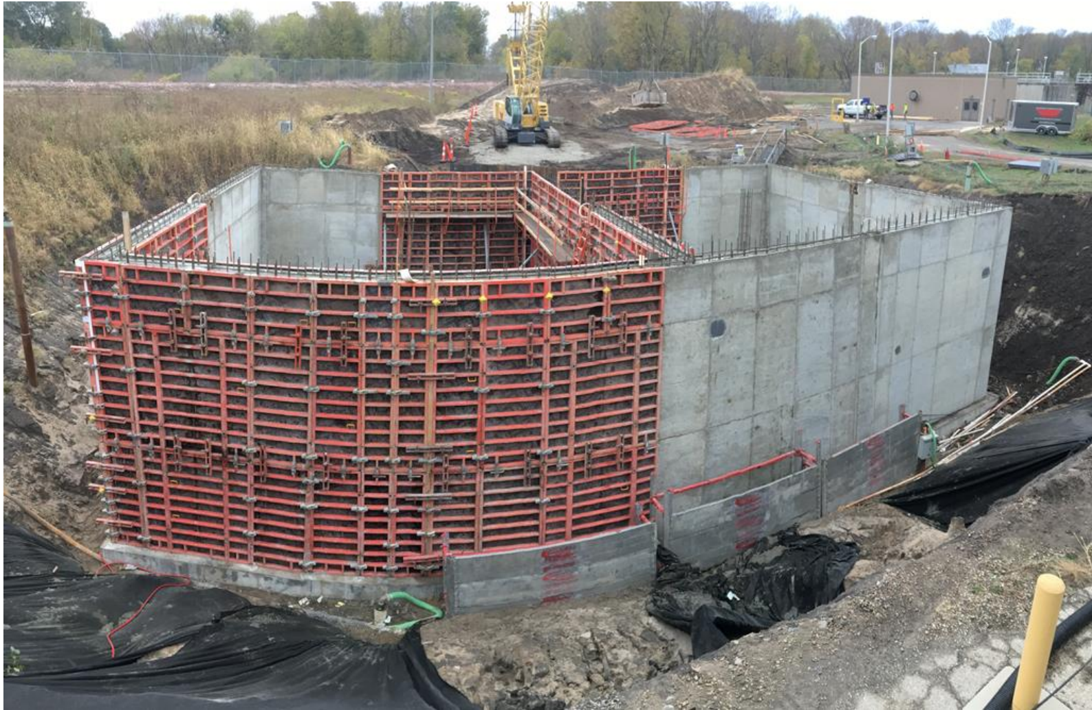
Progress photo – forming walls for centrate tank
