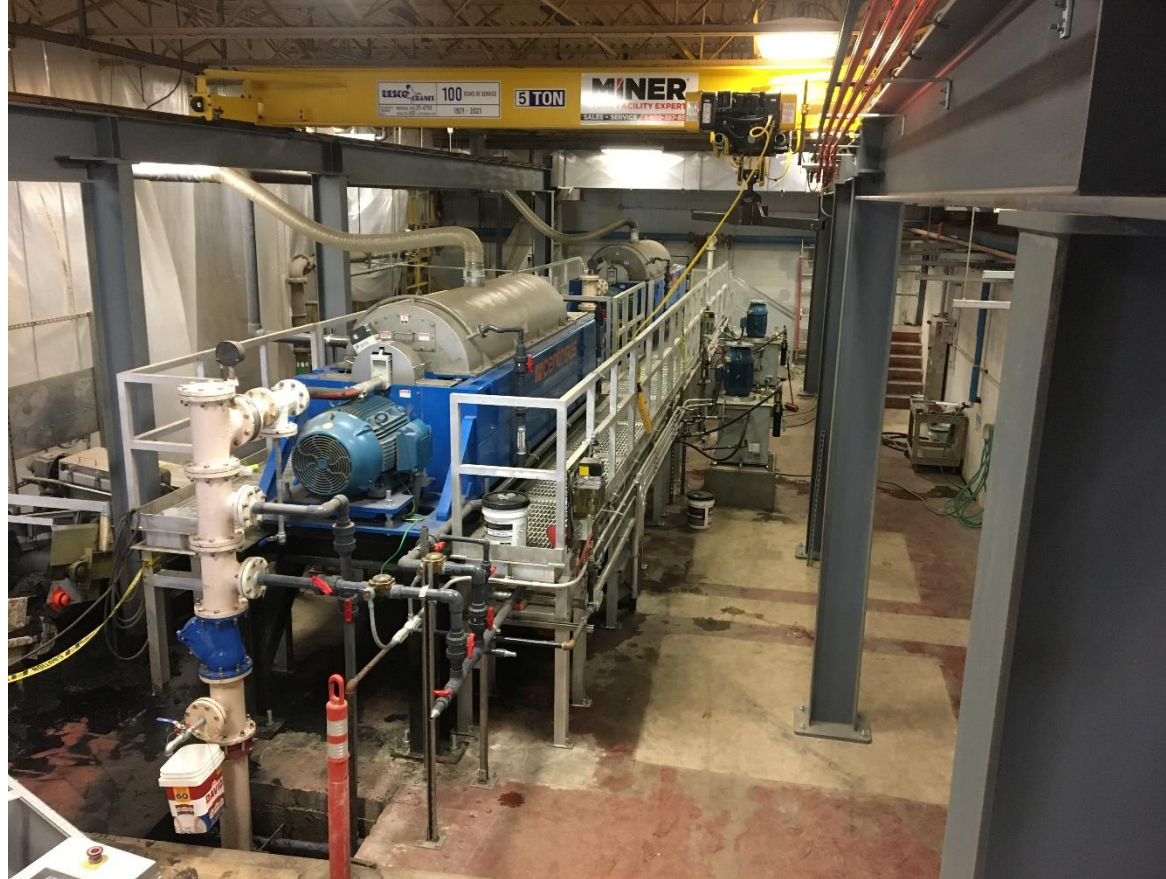
Installation of new centrifuge dewatering equipment in progress
