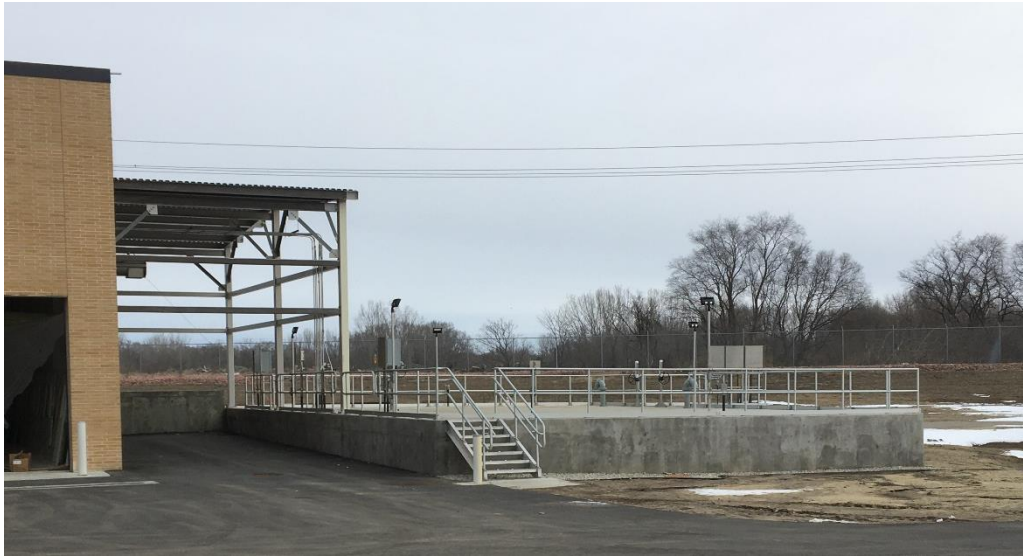
New centrate equalization tank adjacent to the dewatering building
