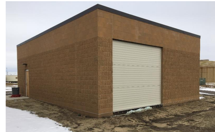
Removable panels allow for future storage tank expansion
